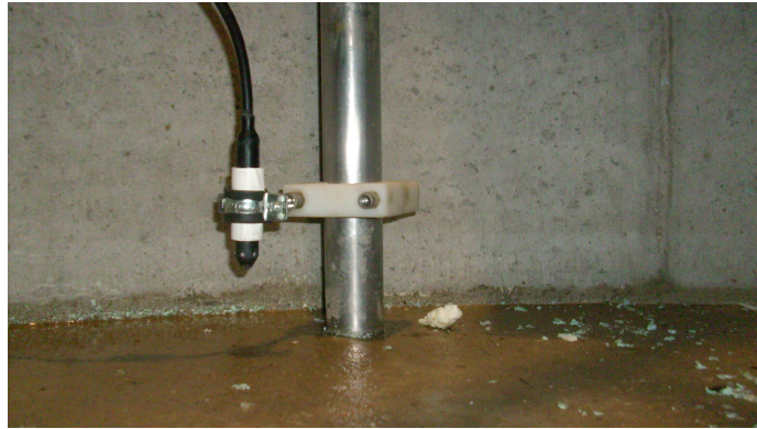
Figure 4.26: Pore pressure transducer placed in the pumping well
