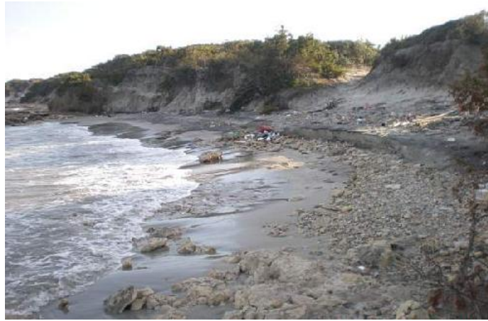
Figure 2.1: Example of coastal erosion at Otranto (LE) - Italy
