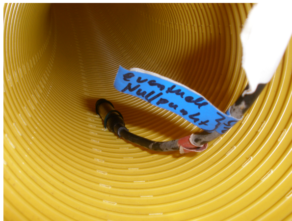
Figure 4.24: Pore pressure transducer inside the drain
