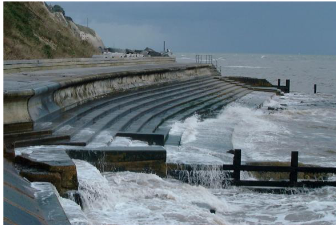
Figure 2.5: Stepped seawall at Wheelers Bay Isle of Wight - England
