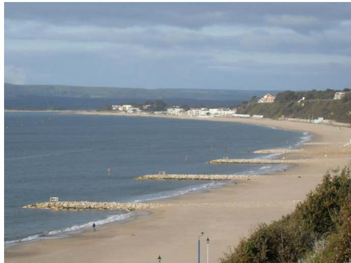
Figure 2.11: Groynes at South of England
