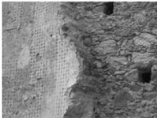
Figure 2: This picture clearly illustrates the use of "Caroselli" as structural element in the wall structure.
