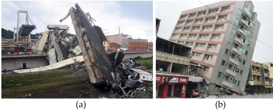
Figure 1. Catastrophic failure of civil constructions: (a) Morandi bridge in Genova - Italy, and (b) civil building in Tainan - Taiwan.
