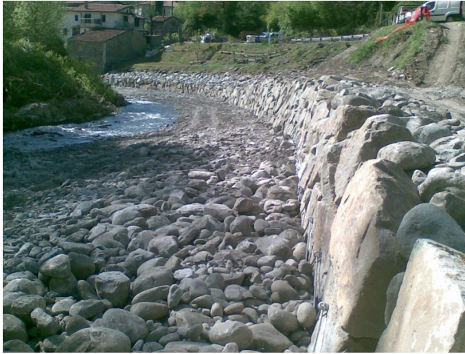
Figure 1.1: Example of erosion protection through coarse-sediments coating in Crespiano Comunita Montana Lunigiana , Tuscany, Italy
